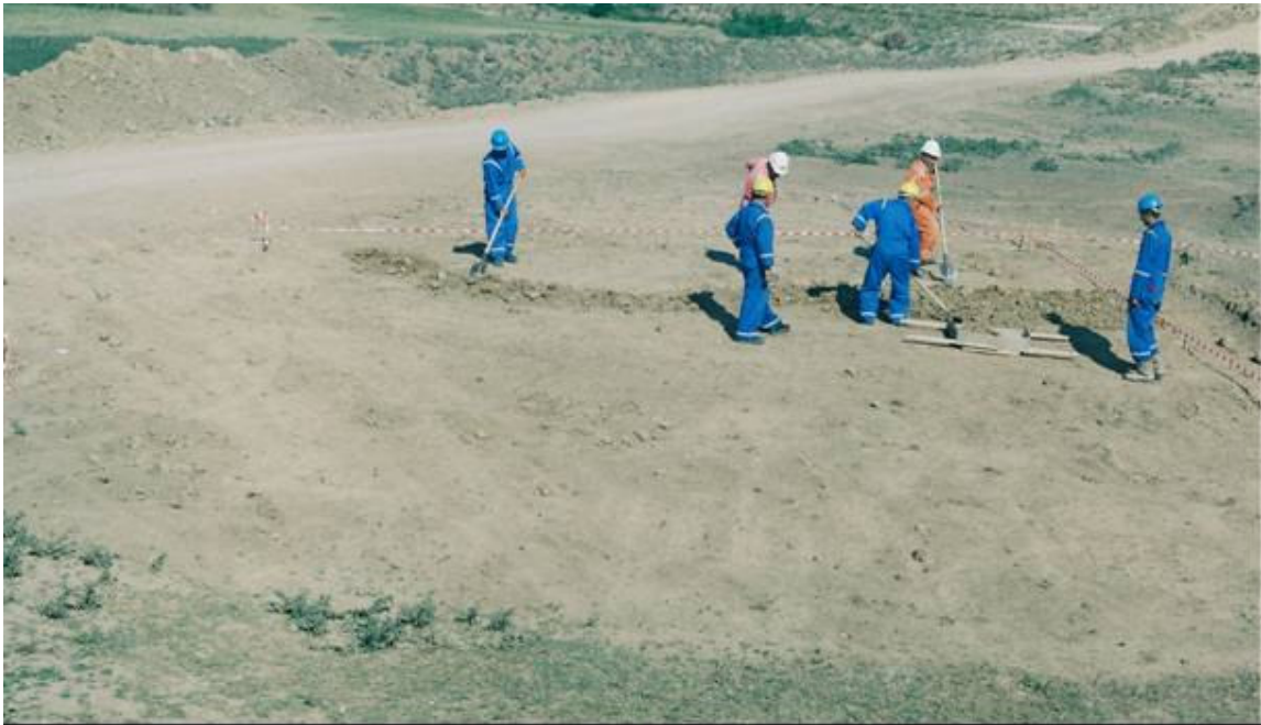
Photo 1. View of the excavation site.
